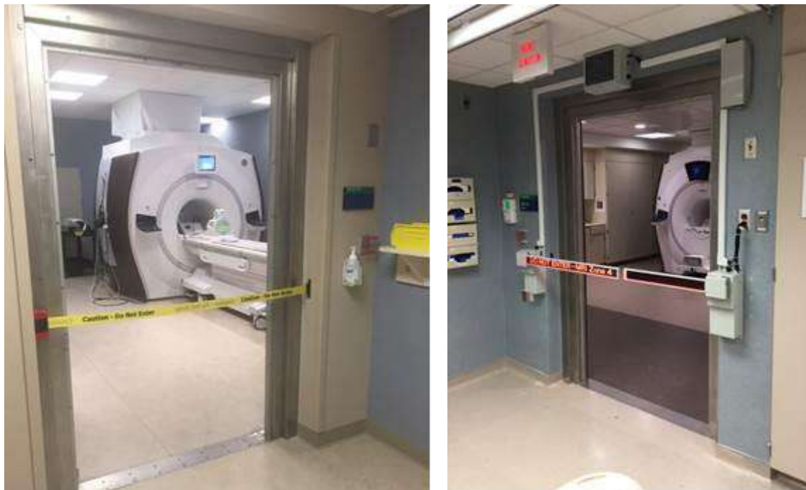
FIGURE 4. Examples of door barriers to Zone IV.
