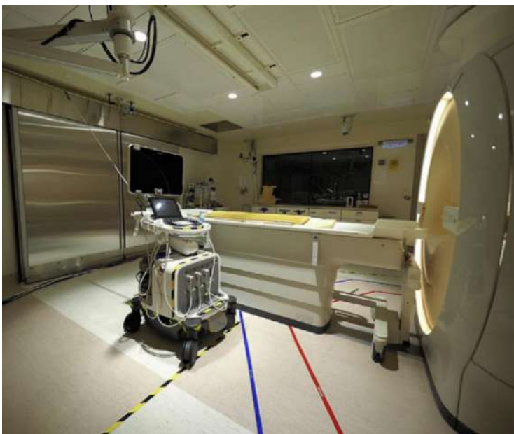
FIGURE 20. Tethering of an appropriately labeled MR Unsafe ultrasound equipment in a hybrid procedural suite, preventing it from crossing the black and yellow striped line. The ultrasound system is positioned beyond the 100-gauss (blue line) and 300-gauss (red line) areas. The intention of the tether is to prevent the ultrasound system from entering a fringe field that would cause it to become a projectile. Extensive physics testing was performed on the ultrasound equipment, verifying its safe location as pictured, prior to its deployment in Zone IV. (Figure used with permission of the Mayo Clinic Foundation for Medical Education and Research, all rights reserved.)
