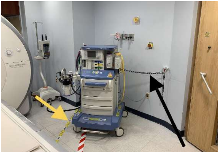
FIGURE 19. Tethering and placement of anesthesia equipment in Zone IV. Note the tether (black arrow) and the 200-gauss line (yellow arrow).
